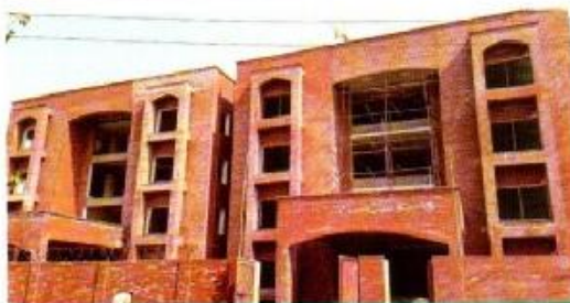
Construction of REC/DEC office Sargodha
