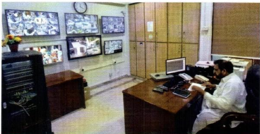
Control room of CCTV surveillance system
