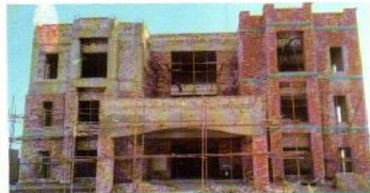
Construction of DEC office Layyah
